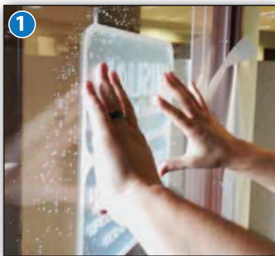
Spray surface with glass cleaner; slide vinyl in place.
